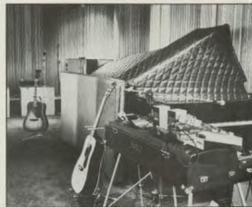
Irregularly shaped wall cavities of slot absorber/diffusers and bass traps
